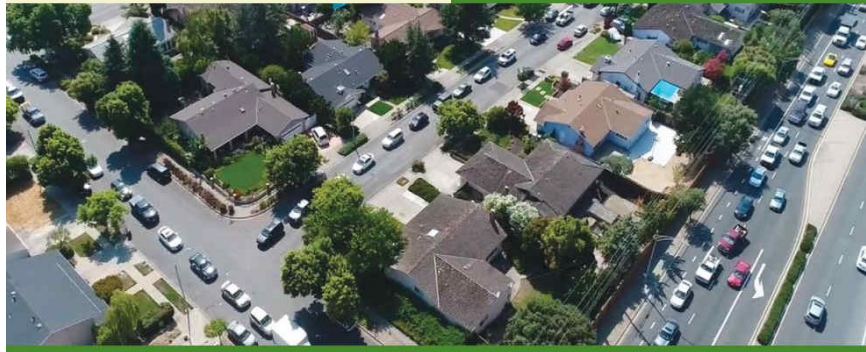
Photograph of a congested Fremont neighborhood near I-680 taken from a drone camera
