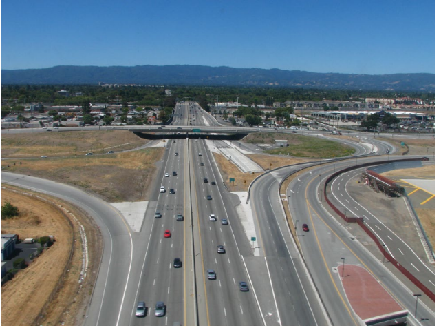
I-880 / Coleman Avenue Interchange
